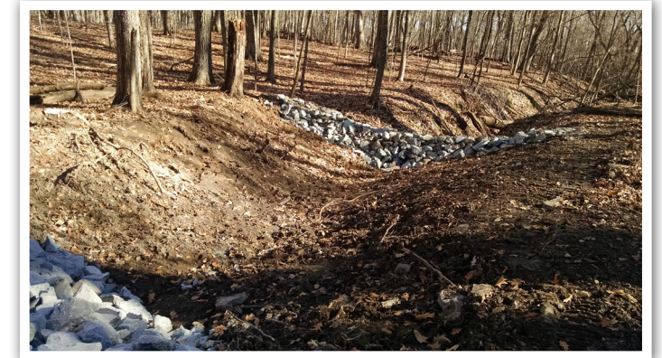
Rock check dams, below the culvert on the opposite side of the driveway, further slow the water preventing erosion in streams that flow to Deer Lake.
