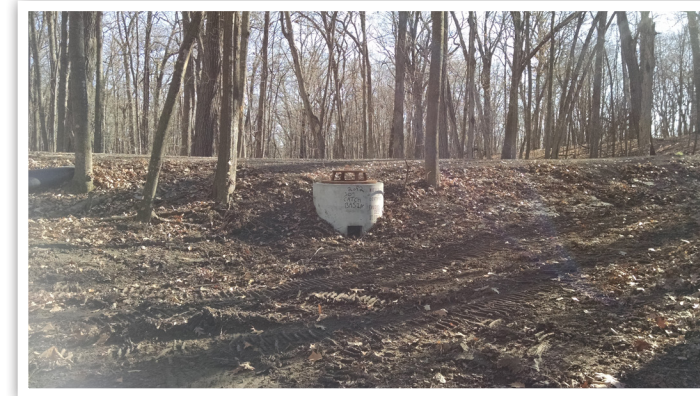
The riser pipe shown above holds back runoff water creating a temporary ponding area above the driveway.
