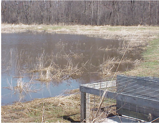
Basin and outlet trash rack
