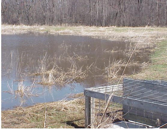
Basin and outlet trash rack
