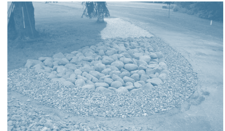
A rock infiltration pit is another way to capture runoff water.
