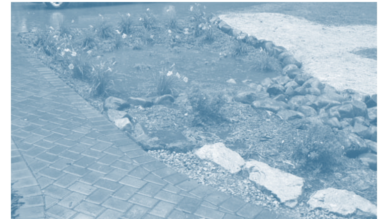
These rain gardens will drain within 12 hours of a storm.
